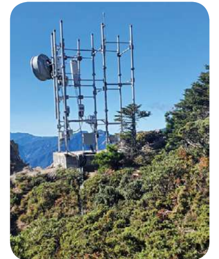
Built mobile communication base station at the Jiaming Lake Cabins to improve signal
